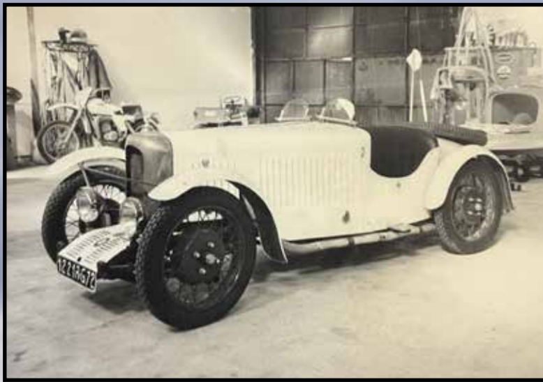
This photo, taken at the home of a collector in the Burgundy region, shows that the car still has its original bonnet, recognisable by the interruption in the bonnet louvres.
